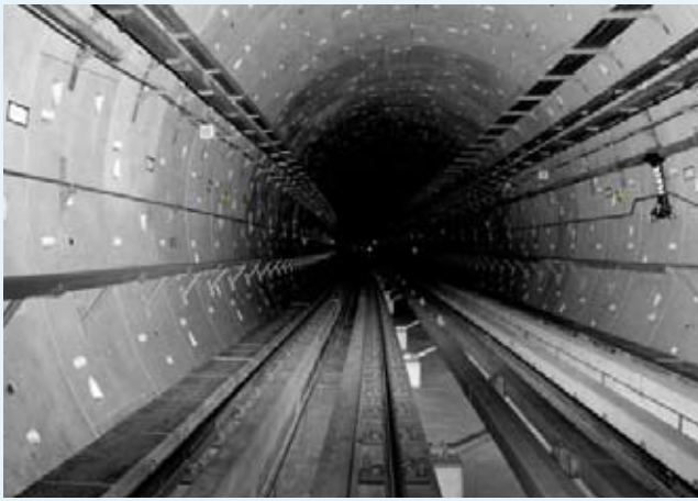
Fig. 9 : Laser Scanning of a Tunnel
