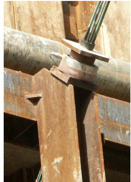
Centre hole load cell installed on anchored sheet pile
